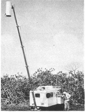
ALL TERRAIN VEHICLE, containing an analyzer, computer, and a detector at the end of a boom, counts radiation on Enewetak. Anti-C suits in the hot, humid climate tended to be uncomfortable.
